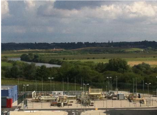
Gas Reception Facility and River Trent
