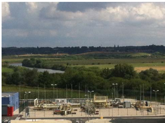
Gas Reception Facility and River Trent
