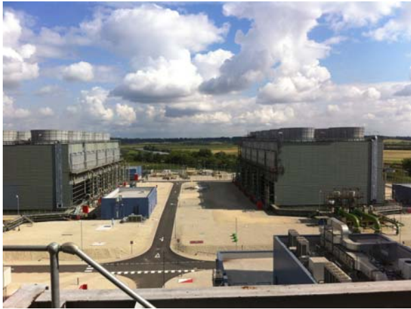
Views of the Cooling Towers
