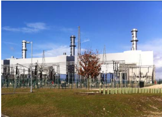
Switch yard connection to the National Grid
