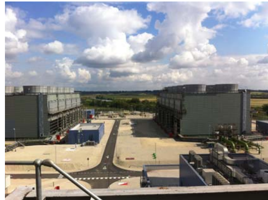
Views of the Cooling Towers
