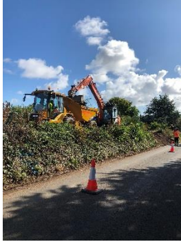
Works to the hedgerow alongside Shurton Road
