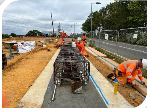
Installation of the retaining wall on the north east corner is in progress.
