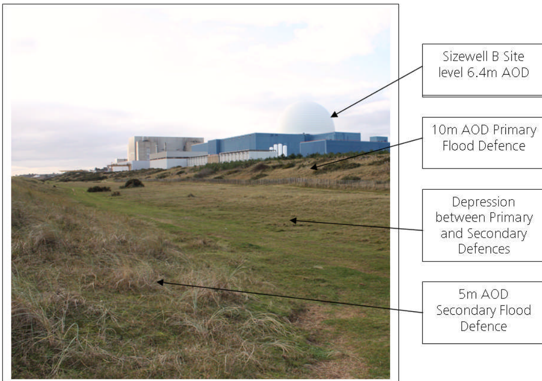
Figure 3.A.3: Sizewell B Flood Defences
