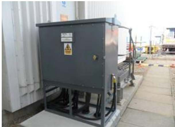
External Connections box for SZB battery charging diesel generator
