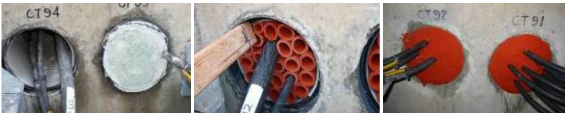
Sealing of Electrical Penetrations, Before and After
