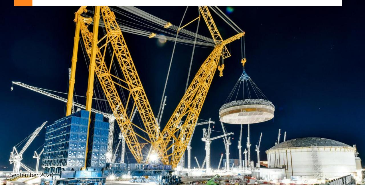
Lifted by the world's largest crane Big Carl, just nine months after the same lift for the first reactor, construction of the 170 tonne liner cup was more efficient than the identical part on Unit 1.
