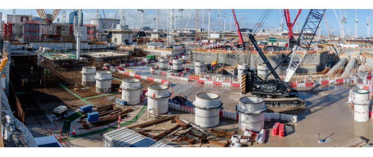
In April, Socea Denys, completed the installation of Unit 1's CRF pipes. They will channel cooling water into the power station.
