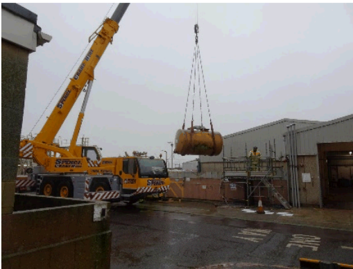
Figure 4. Removal of diesel storage tank
