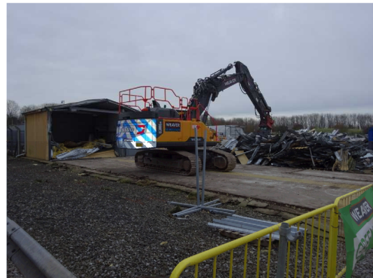
Figure 5. Segregating waste material from the demolition of temporary buildings
