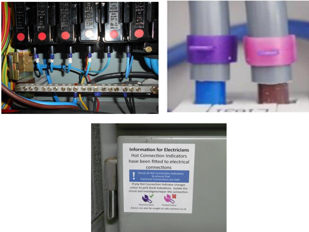
Figure 3.1: Cable hot connection indicators
