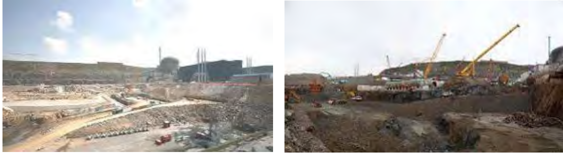
Figure 4.2: Site Preparation Works (Flamanville 3 - France)
