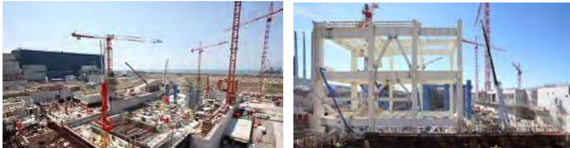
Figure 4.3: Construction of Buildings (Flamanville 3 – France)
