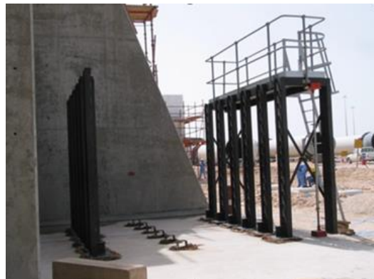
Plate 3-2: Example of a toaster-style storage rack from Flamanville 3
