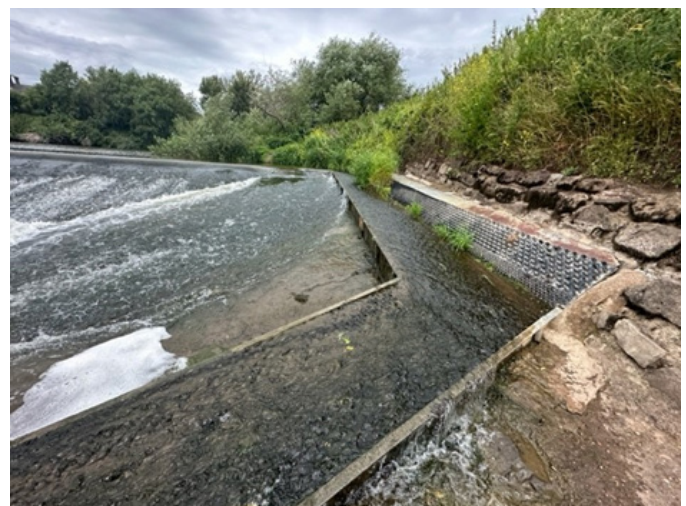
Figure 4 The tidal limit of the River Severn at Upper Lode Weir near Tewkesbury. Right panel shows the current fish pass.
