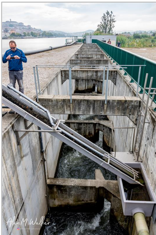
Figure 7 The Coimbra Dam Vertical Slot Fish Pass. Photograph by Dr A.M. Walker, October 2018.
