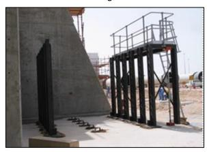
Figure 13 - Example of a toaster-style storage structure from Flamanville 3
