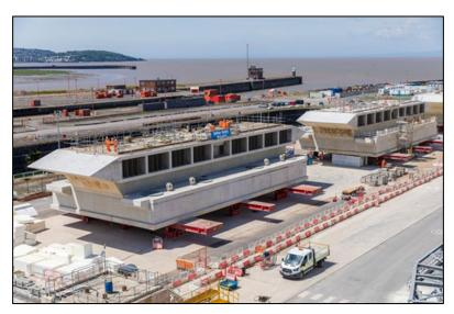
Figure A3-3 -Hinkley Point C's LVSE intake heads are specially designed to reduce the speed at which water is fed into the cooling system
