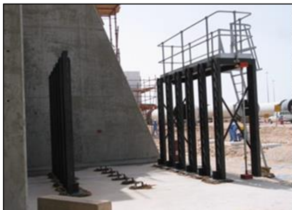
Figure 13 – Example of a toaster-style storage structure from Flamanville 3
