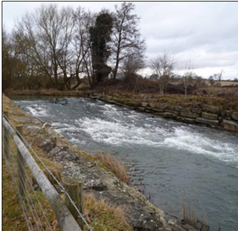
Figure 26 - Mousenatch Weir © Environment Agency
