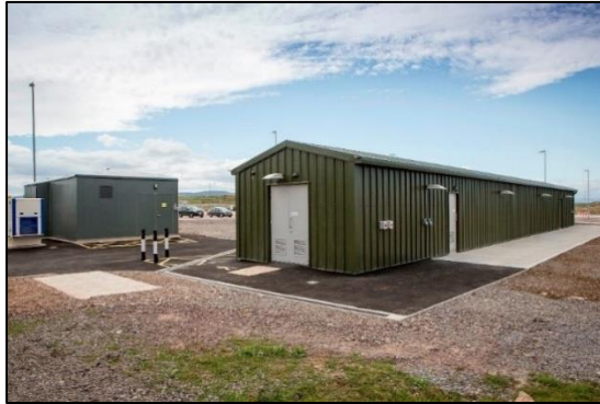
Figure 11 – Photograph of the existing Electrical Substation at HPC
