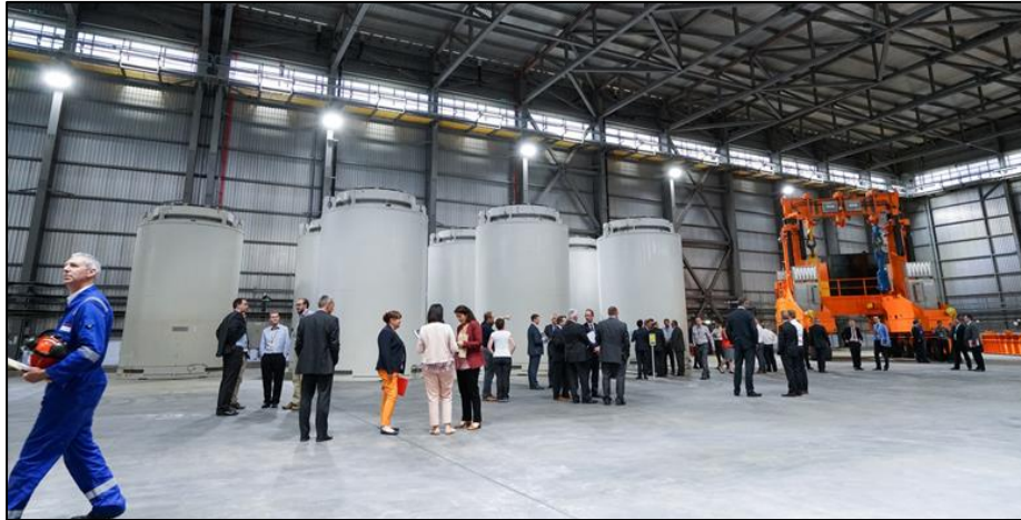
Figure 7 - The 'dry' ISFS at Sizewell B power station
