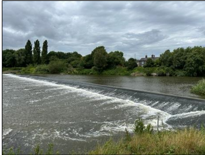
Figure 23 - Upper Lode Weir on River Severn
