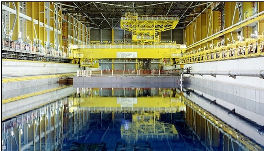
Figure 6 - The 'wet' ISFS at Sellafield
