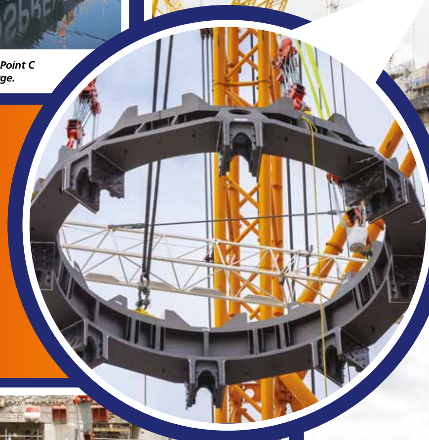
The support ring (inset) was craned over the reactor building and lowered into place in a meticulous operation.
