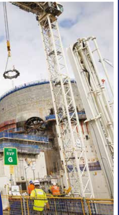
The support ring (inset) was craned over the reactor building and lowered into place in a meticulous operation.
