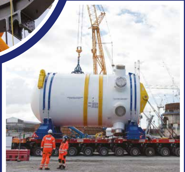
The Reactor Pressure Vessel, which has already arrived at Hinkley Point C, will be installed on top of the support ring.
