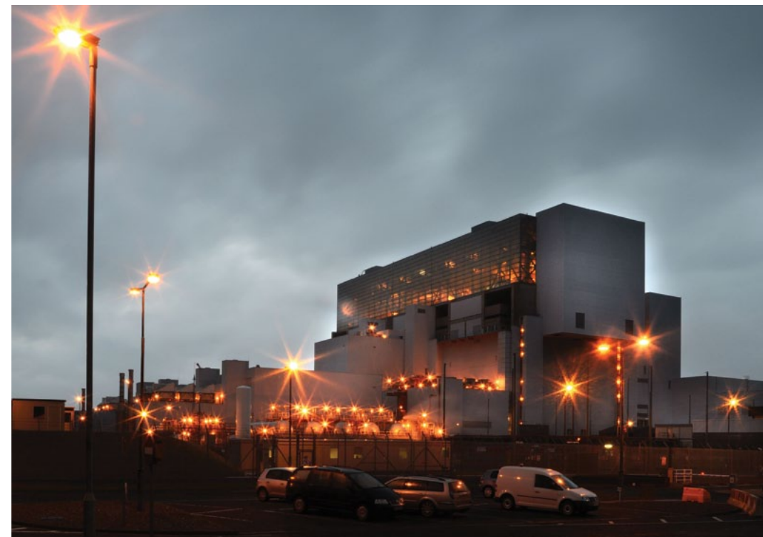
Hunterston Power Station
