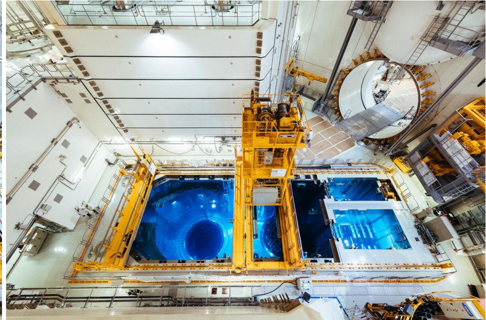
Above: Reactor pressure vessel cavity both empty, and filled with water at Olkiluoto 3 in Finland
