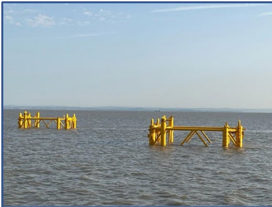
Photo showing example of metal frames (HAF's) exposed and visible at low water.
