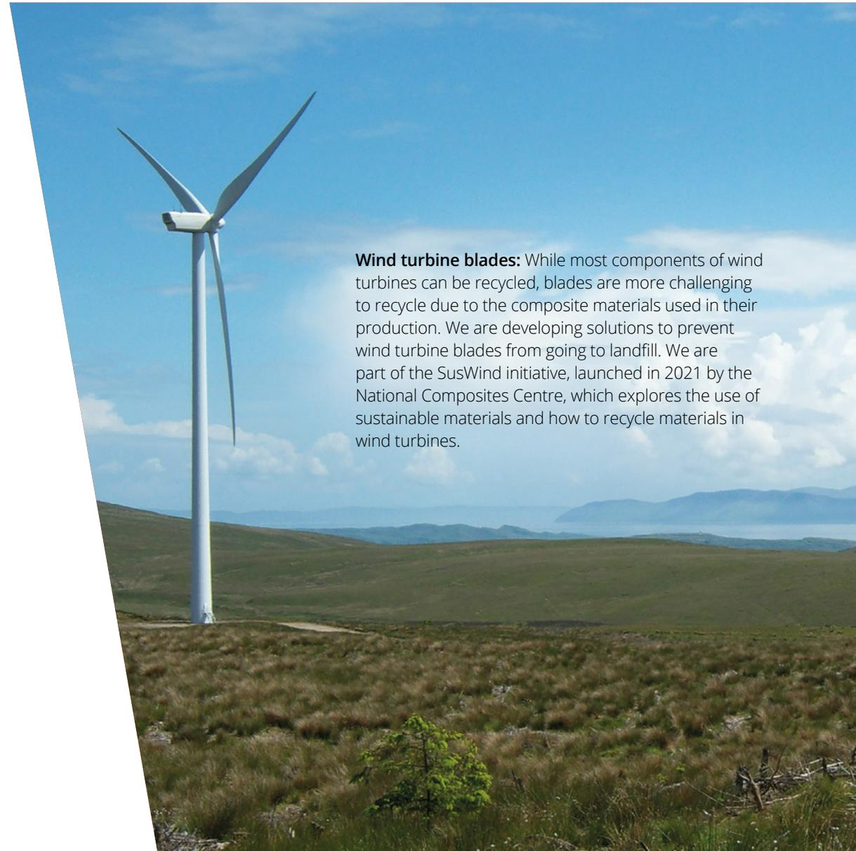
**Wind turbine blades:** While most components of wind turbines can be recycled, blades are more challenging to recycle due to the composite materials used in their production. We are developing solutions to prevent wind turbine blades from going to landfill. We are part of the SusWind initiative, launched in 2021 by the National Composites Centre, which explores the use of sustainable materials and how to recycle materials in wind turbines.
