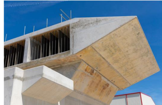
The design of the intake heads reduces the speed of the water being taken into the cooling pipes and are installed sideways to the tidal flow in the Severn Estuary. This reduces the risk of fish entering the pipes.
