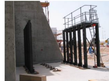
Example of a toaster-style storage rack from the Flamanville 3 nuclear power station in France.
