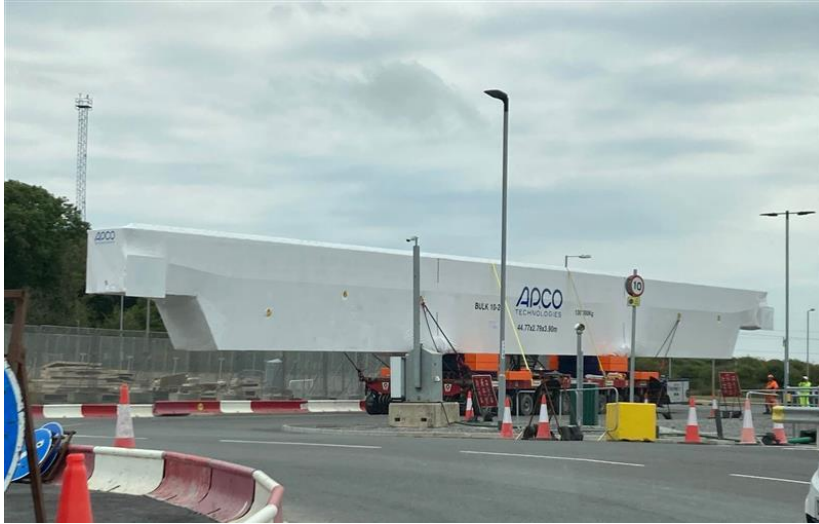
Polar crane beam
