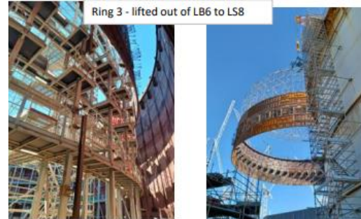
Unit 1 – Liner Ring 3 lift
