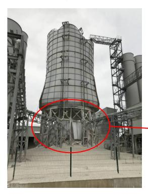
The silo was erected in June 2018 as a temporary works structure used in construction and was not a permanent part of the power station. The silo was of a bolted design with welded flanges, as opposed to lap joints. The main cylinder was installed in five ring sections, each three panels in height (28 individual panels per ring). The cone/hopper section was manufactured in three sections; a transition section (18 panels) and upper cone/lower cone sections (36 panels each).
