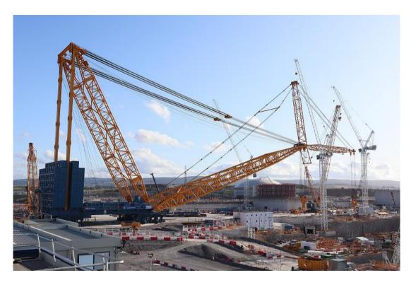
Standing at 250 metres tall, it is taller than the London Eye and the Statue of Liberty. It has 52 counter weight containers each weighing 1000 tonnes, and is supported on 96 wheels travelling along a specially designed track.
