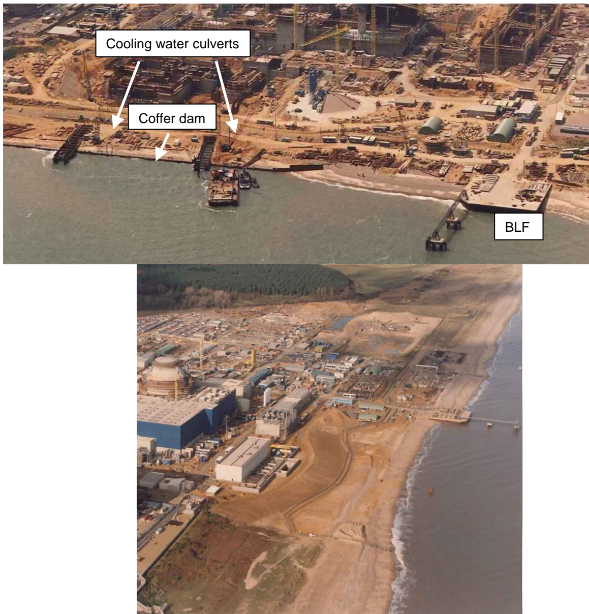
Figure 25: Aerial photographs of the coast during Sizewell B construction. Oblique aerial photograph looking west, showing details of the beach landing facility (BLF) on the right and the intake and outfall culverts on the left (May 1990). Note the removal of the beach and replacement with coffer dam at a position landward of the adjacent shoreline. The resulting bay is likely to be the result of dredging for the cooling water culverts. Bottom: North looking aerial photography (November 1992) following removal of the culvert coffer dam showing the partly constructed sea defences and the embayment formed at the position of the coffer dam and in the lee of the BLF.
