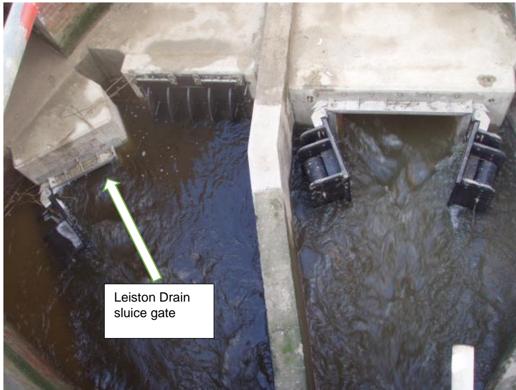
Figure 12: Internal arrangement of Minsmere sluice from “Minsmere sluice update - work now complete” (RSPB, 2014).
