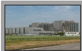
Reactor Generation: Gen-I Type: Magnox Installation: 1956 – 1971 Shut down: 2003 – 2015 Capacity: 200 – 980 MWe
