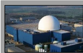
Reactor Generation: Gen-III Type: PWR Installation: 1988 Shut down: 2035+ Capacity: 1250+ MWe
